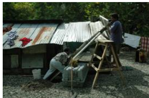
Figure 2 Rotten wooden support eventually fell. No damage - this time.
