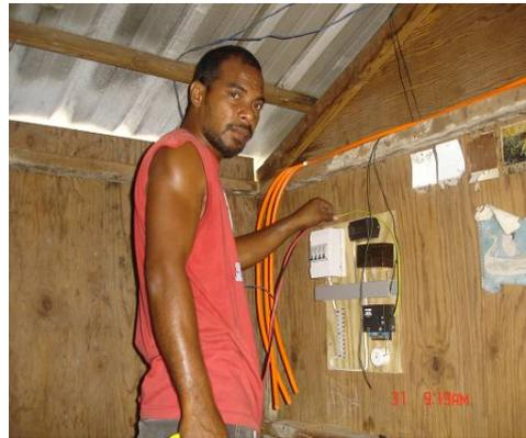
For more than two months MEC staff worked on assembling components into the battery boxes to save time on site. Mounting boards and the charge controllers were preinstalled and system cables pre-cut with terminations made based upon the measurement made during the sample installations. The household controls were also pre-mounted on plywood backing ready for installation.
