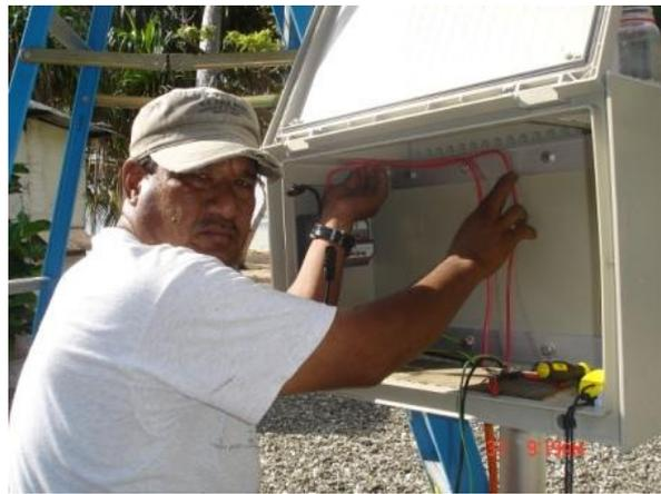
As systems were completed they were left for several days to allow for system checks and for the batteries to gain additional charging with a prolonged trickle charge period. Once the checks had been performed and approved then the system was switched on and the operating procedures / restrictions were explained to the occupants of the house.
